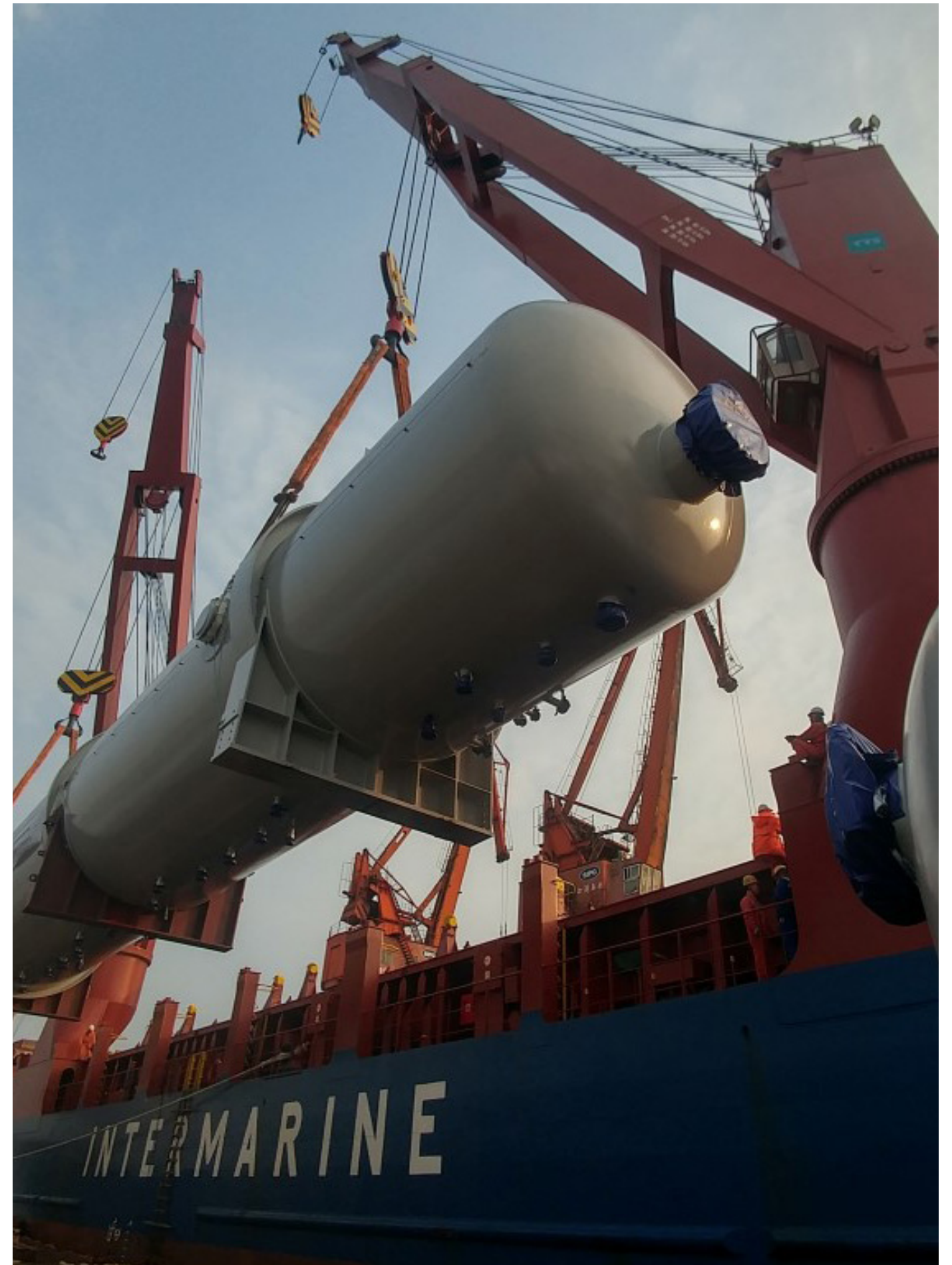
Figure 13: HLV self loading from barge in Shanghai
