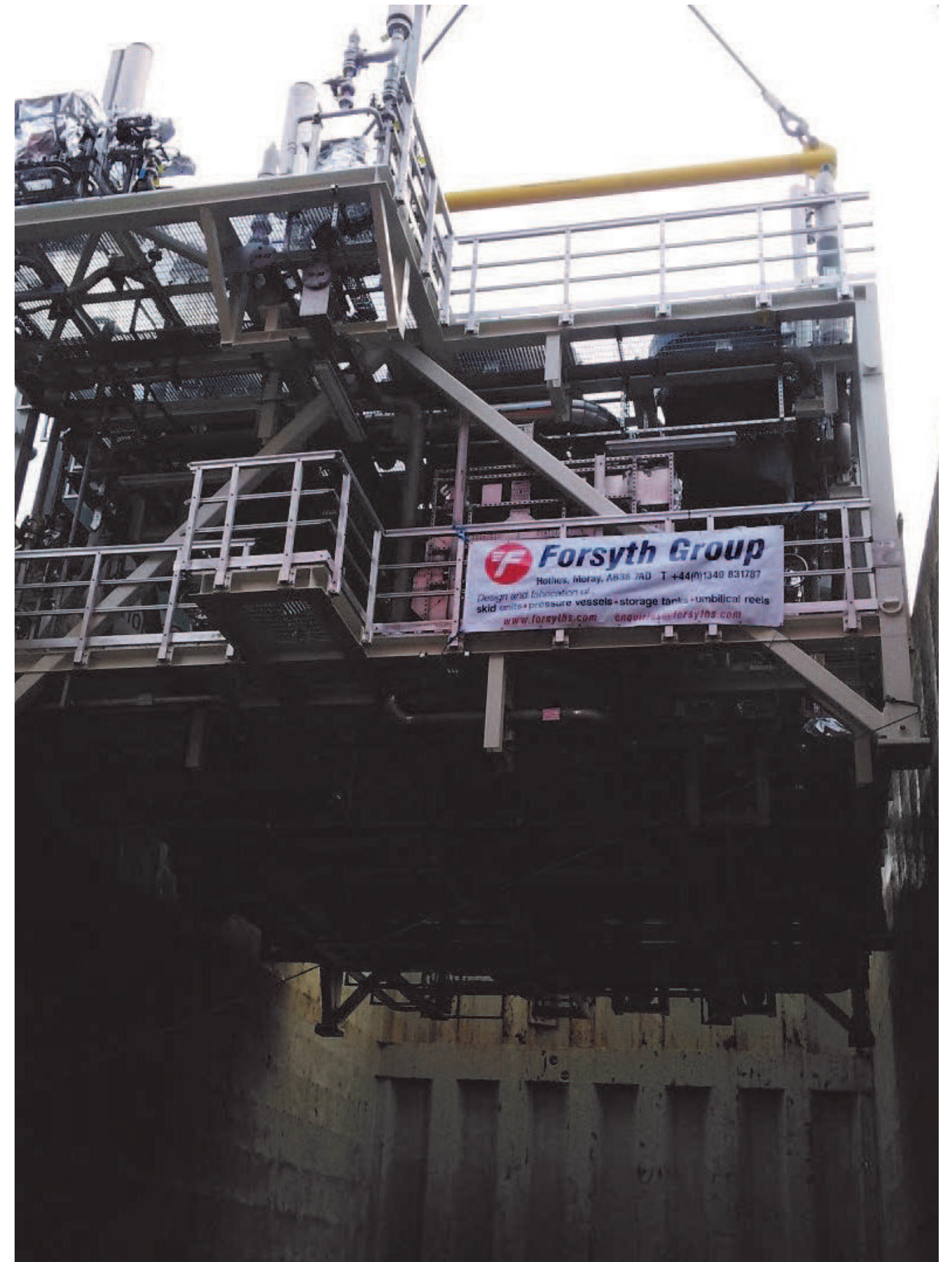
Figure 5: UF Skid being Loaded at Buckie
