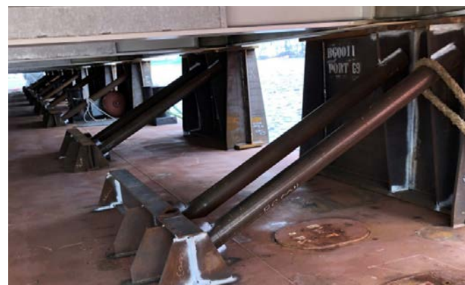
Figures 6-9 (L-R): Typical Module Loadout (Ro-Ro); Pressure vessel on trailer on quayside; Pressure vessel on barge deck departing port; Welded Seafastening
