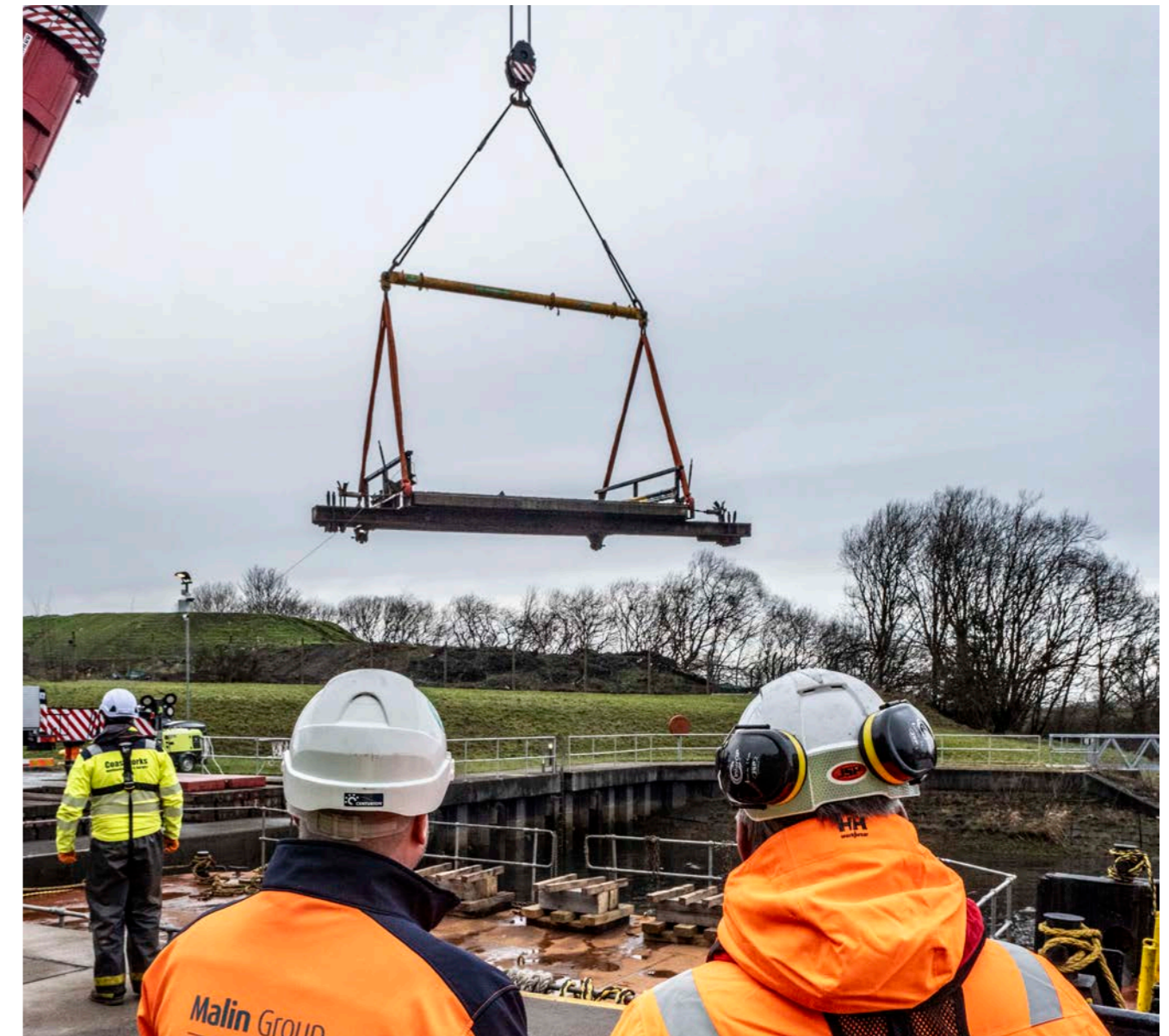
Figure 2: Lift of cargo at quayside
