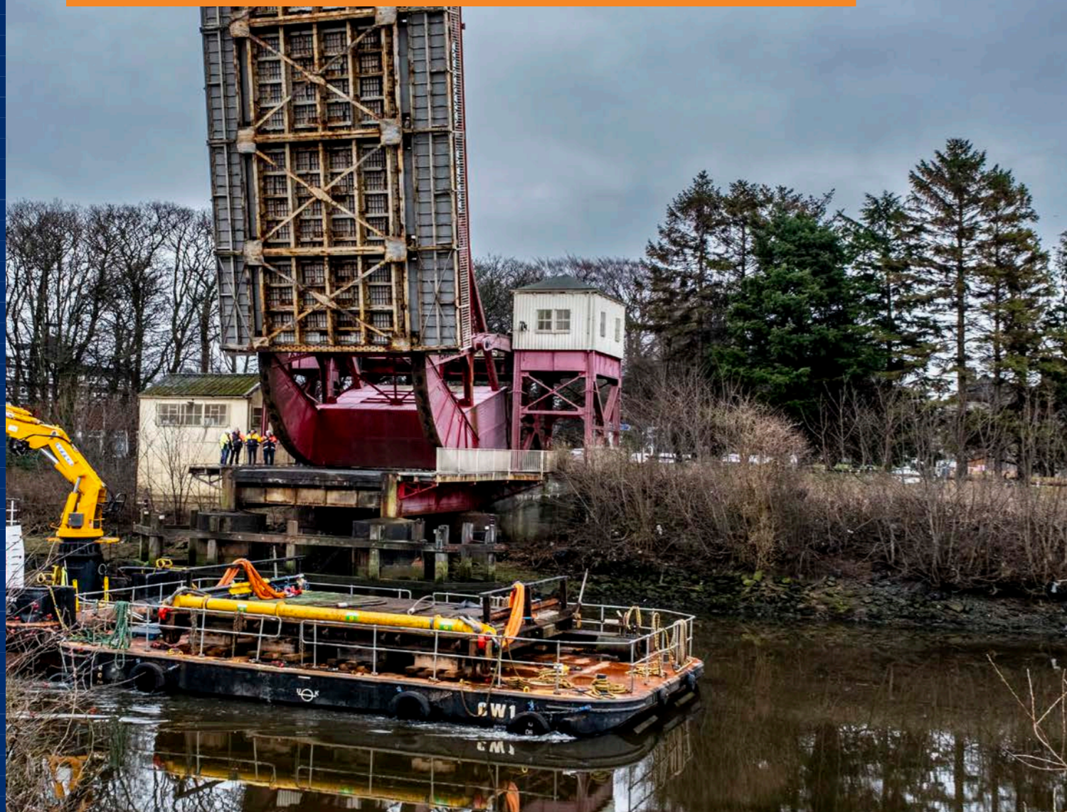
Figure 1: Linkspan in transit on the Whitecart.
