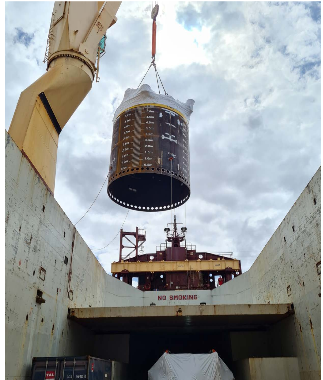
Figure 4: Subsea Manifold Closed Caisson Foundation (CCF)
