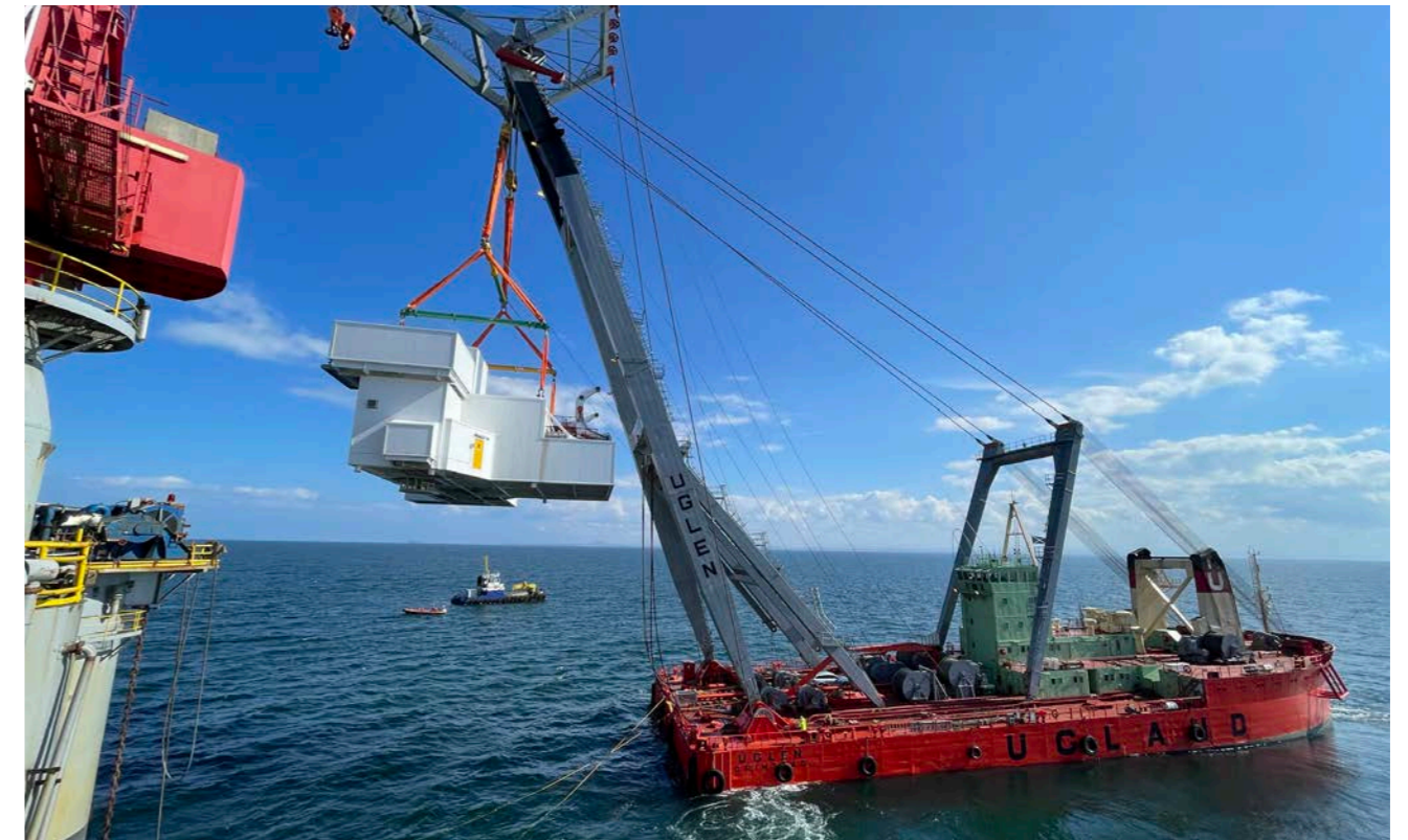
Figure 9: SDS module arriving at the Well-Safe Guardian for installation
