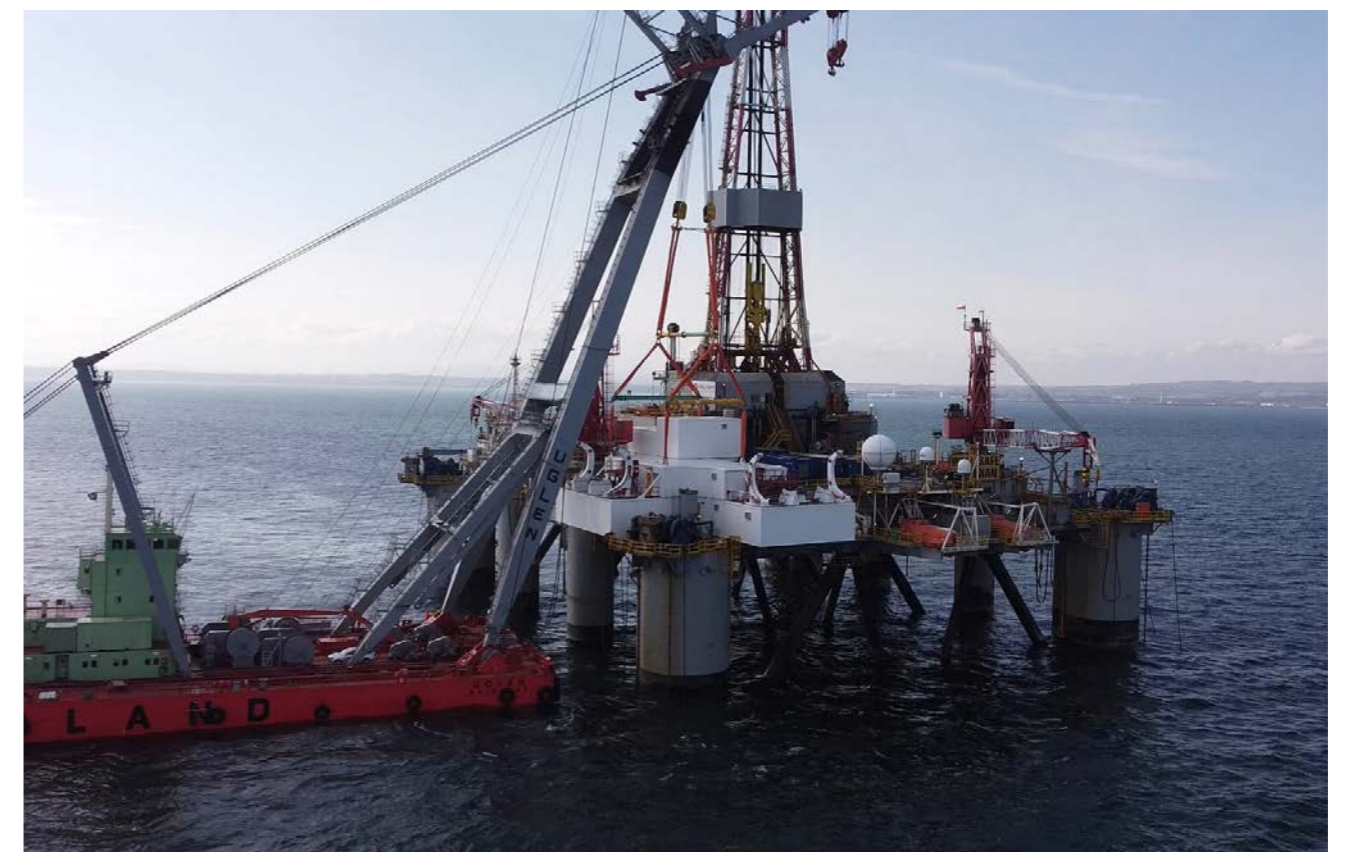
Figure 10: Lifting SDS Module into position on the Well-Safe Guardian
