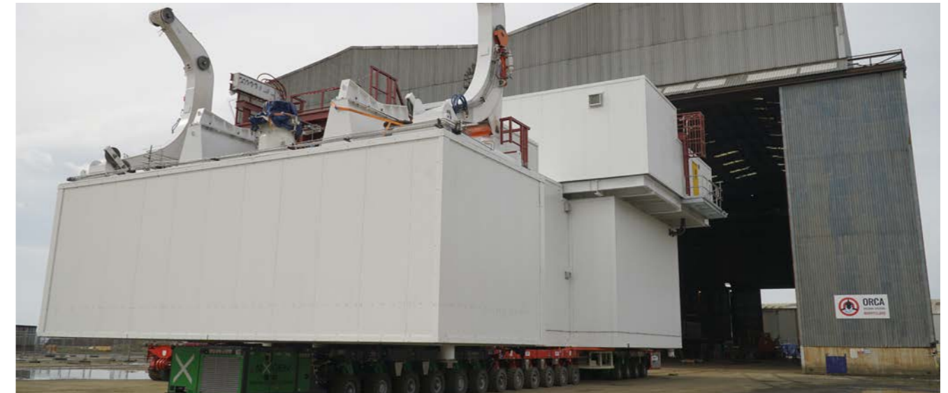
Figure 2: SDS module leaving Burntisland facility on SPMT's, heading for load-out
